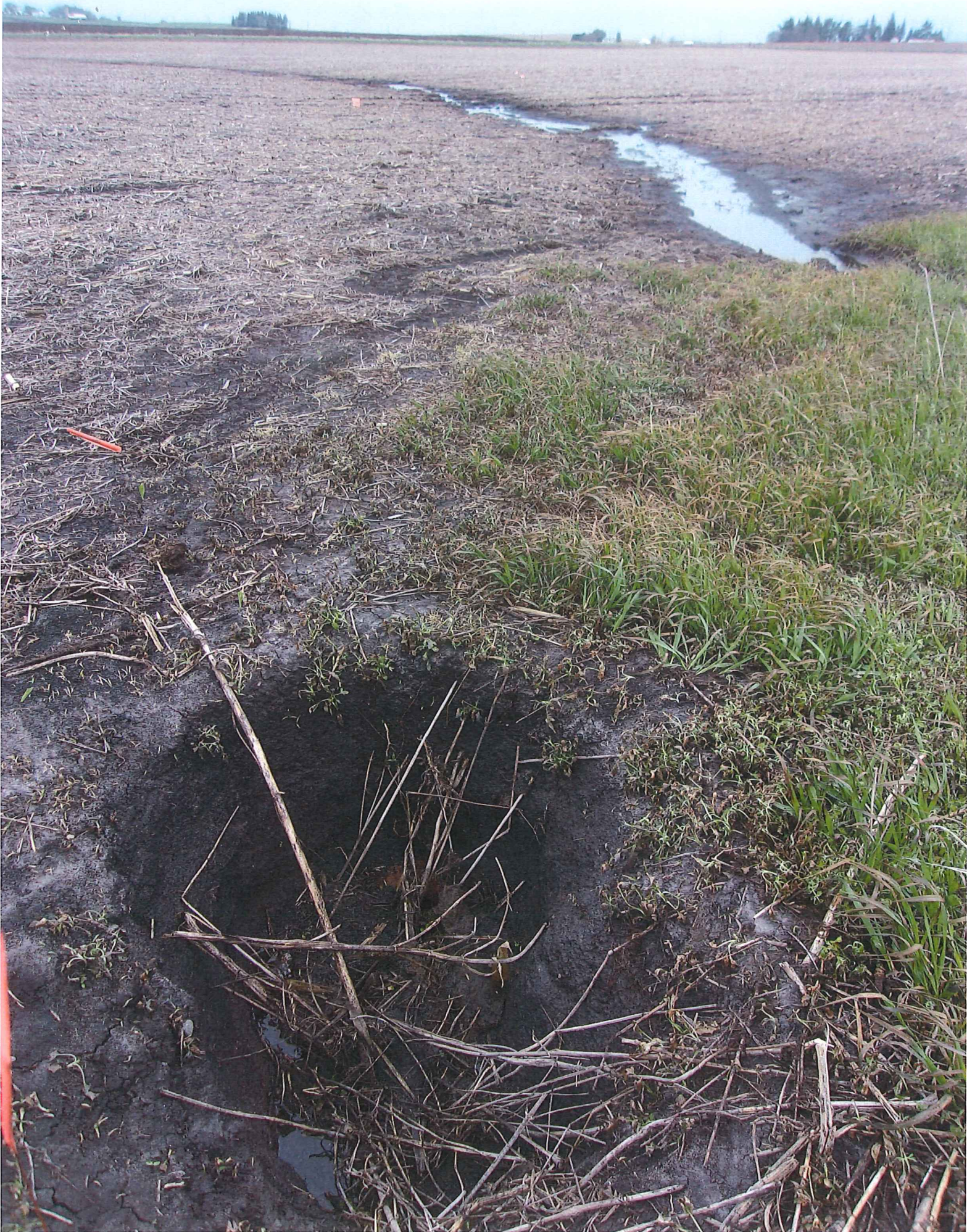
Looking NW @ Biggest Hole, 2' cover
