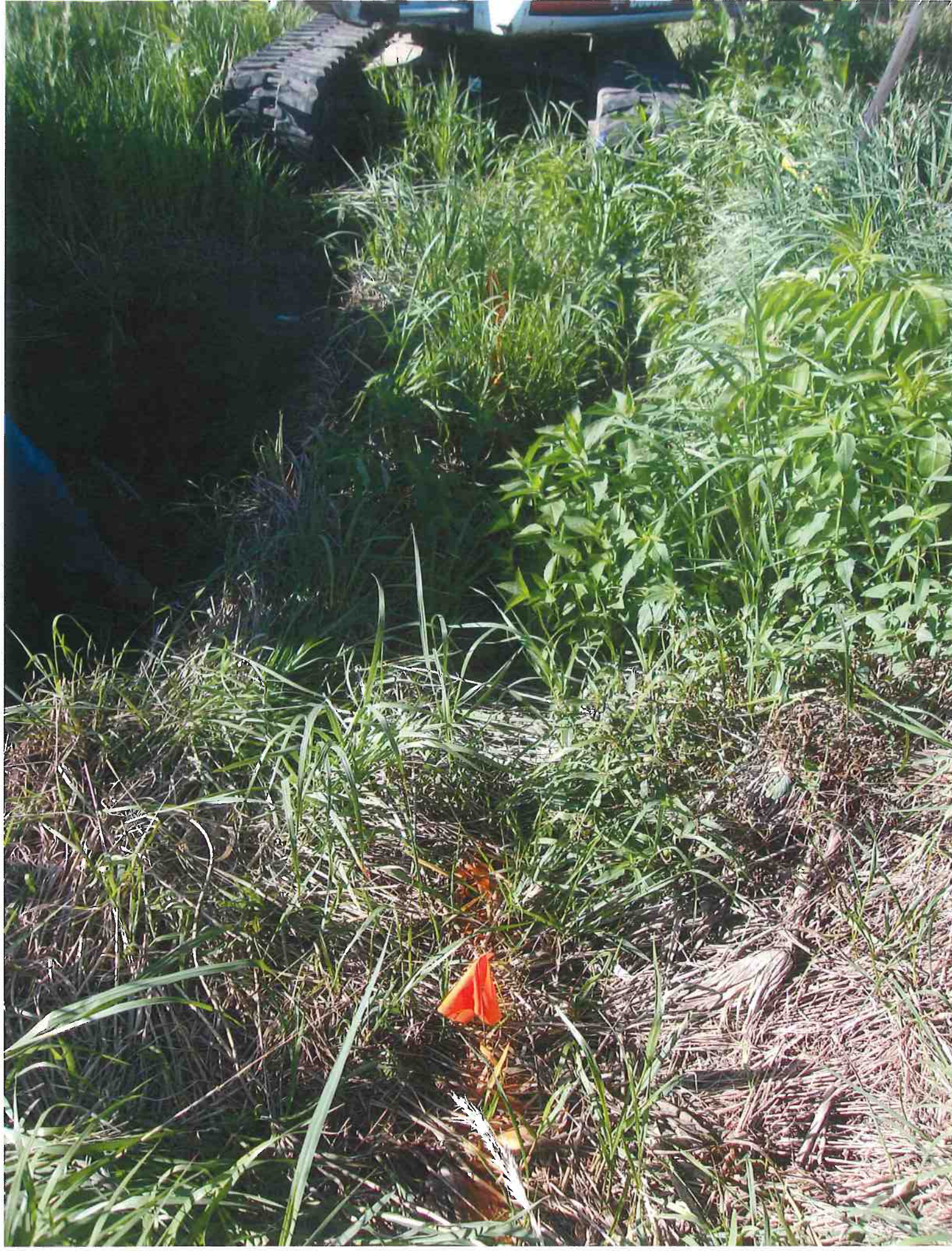
CABLE LOCATES IN DITCH
