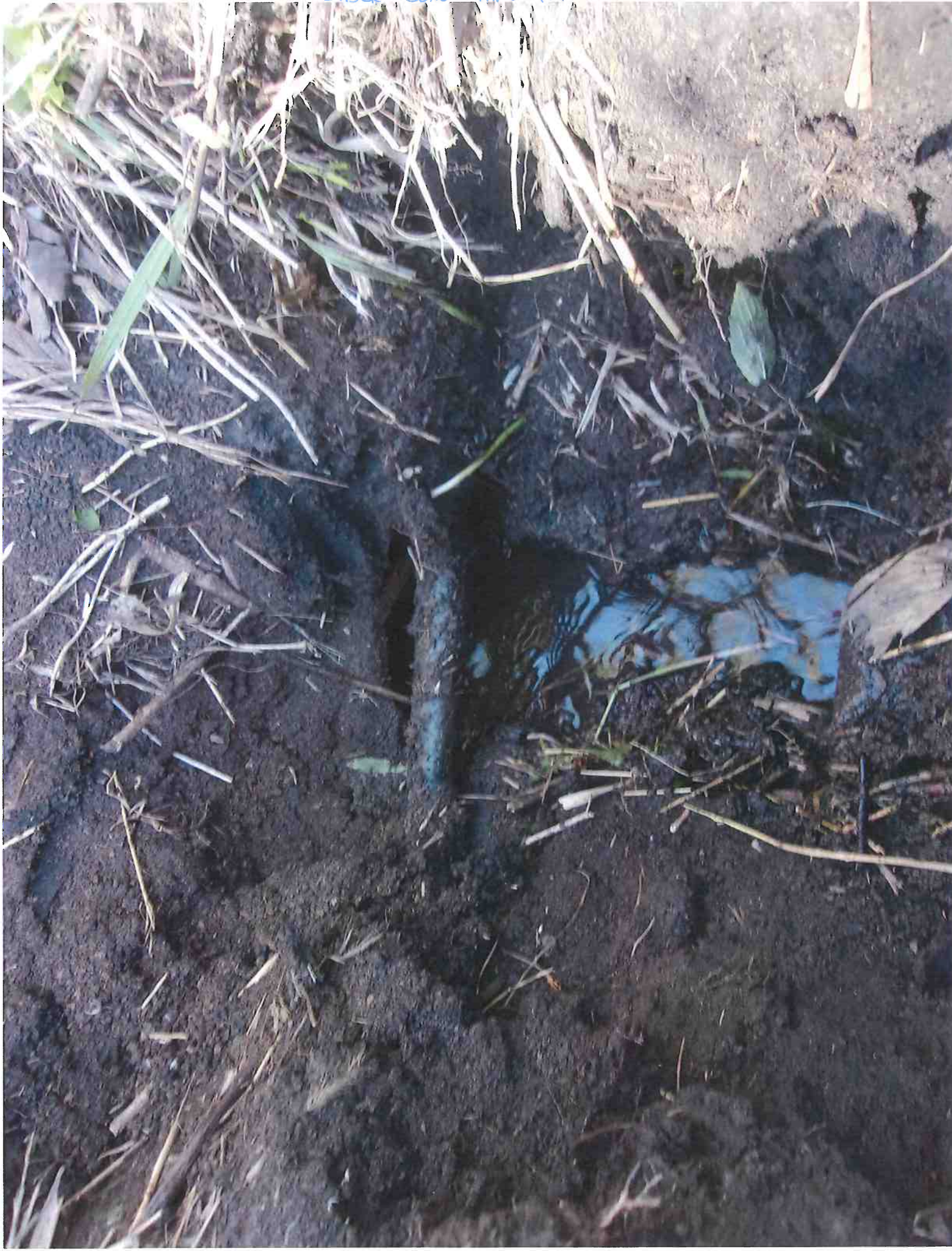
CABLE GOING THRU TIE
